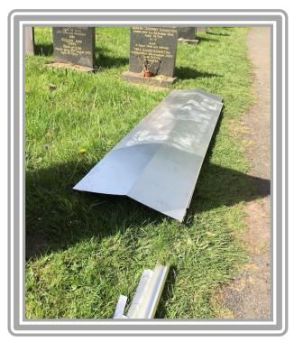
With the roof timbers repaired, on 13 May 2019, it was time for the 'steelmen' from Warren & Neale to start on the new terne-coated stainless steel roof. The steel arrived on site in rolls which were transformed into flat sheets, ridges, and baton rolls using a steel former.
